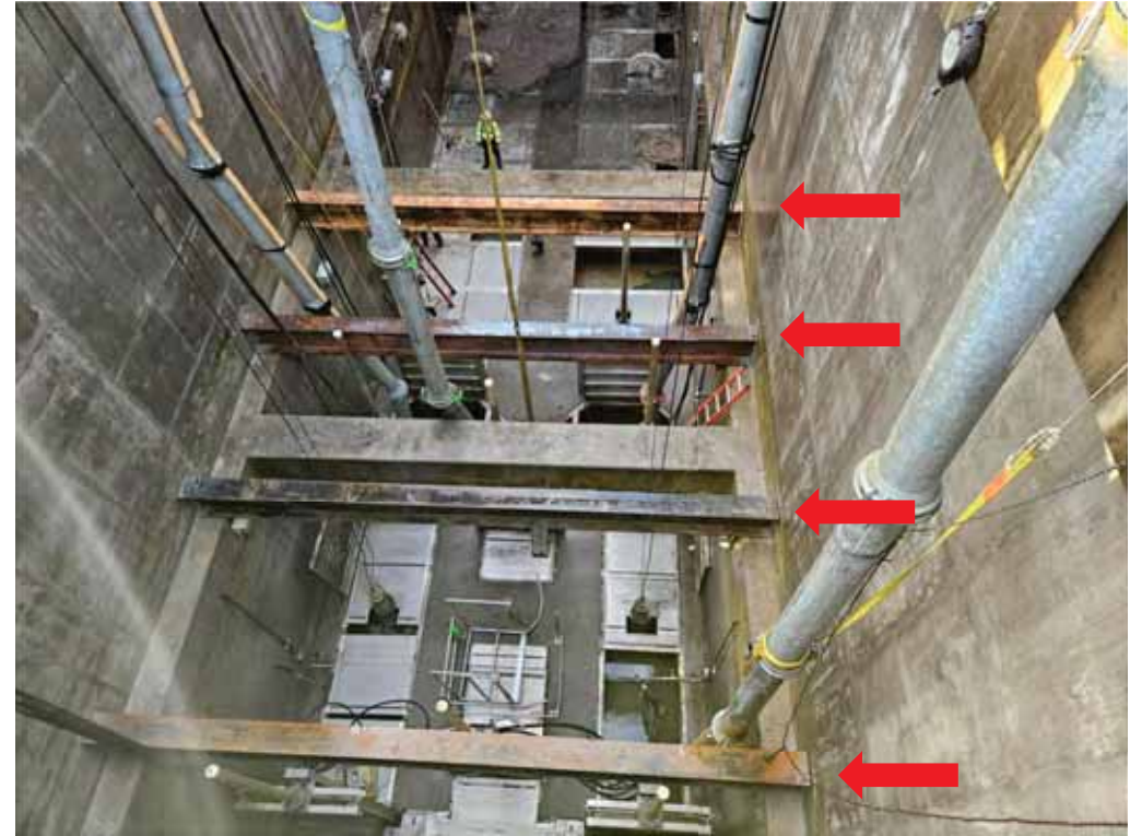
Installation of 4 Mid-Level Support Steel Beams
