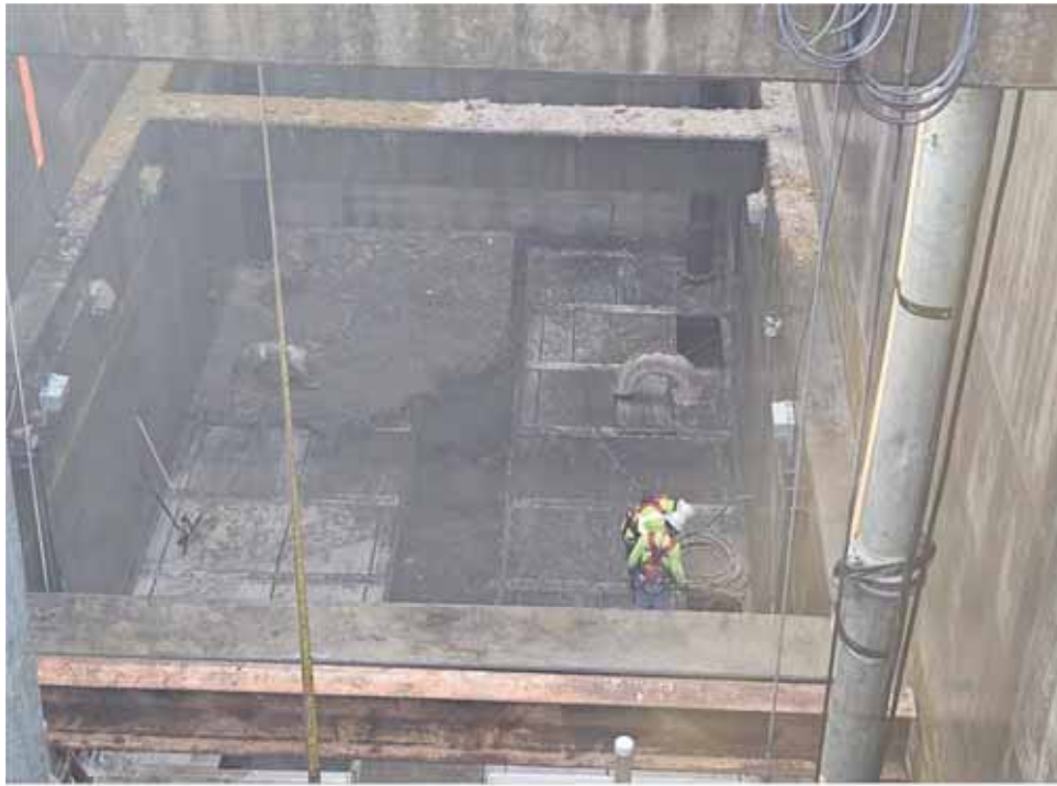
Hot Water Steam Cleaning of Wet Well and Fall Protection Installation
