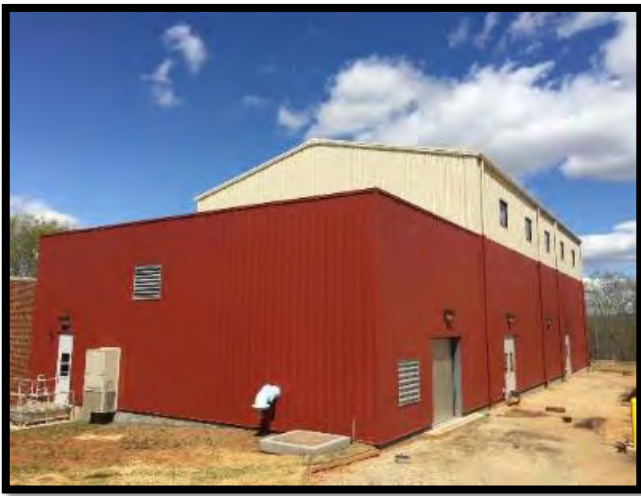
South Rivanna WTP 8 Contactors 320,000 pounds of GAC 8 MGD Capacity
