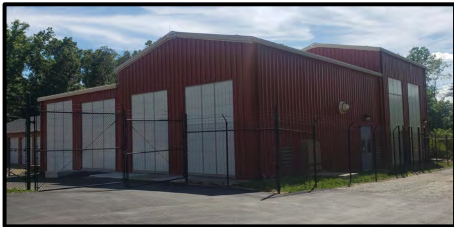
Crozet WTP 2 Contactors 40,000 pounds of GAC 1 MGD Capacity
