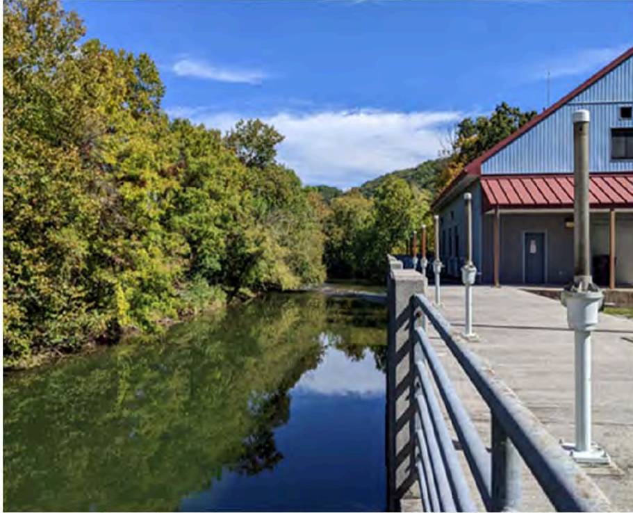
Roanoke River Intake Station
