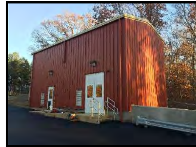
Scottsville WTP 2 Contactors 12,000 pounds of GAC 0.25 MGD Capacity
