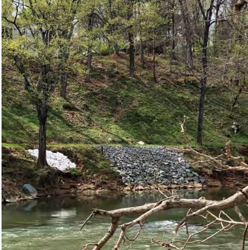
This area near Darden Towe Park required emergency repairs with riprap when erosion exposed utility lines in 2019
