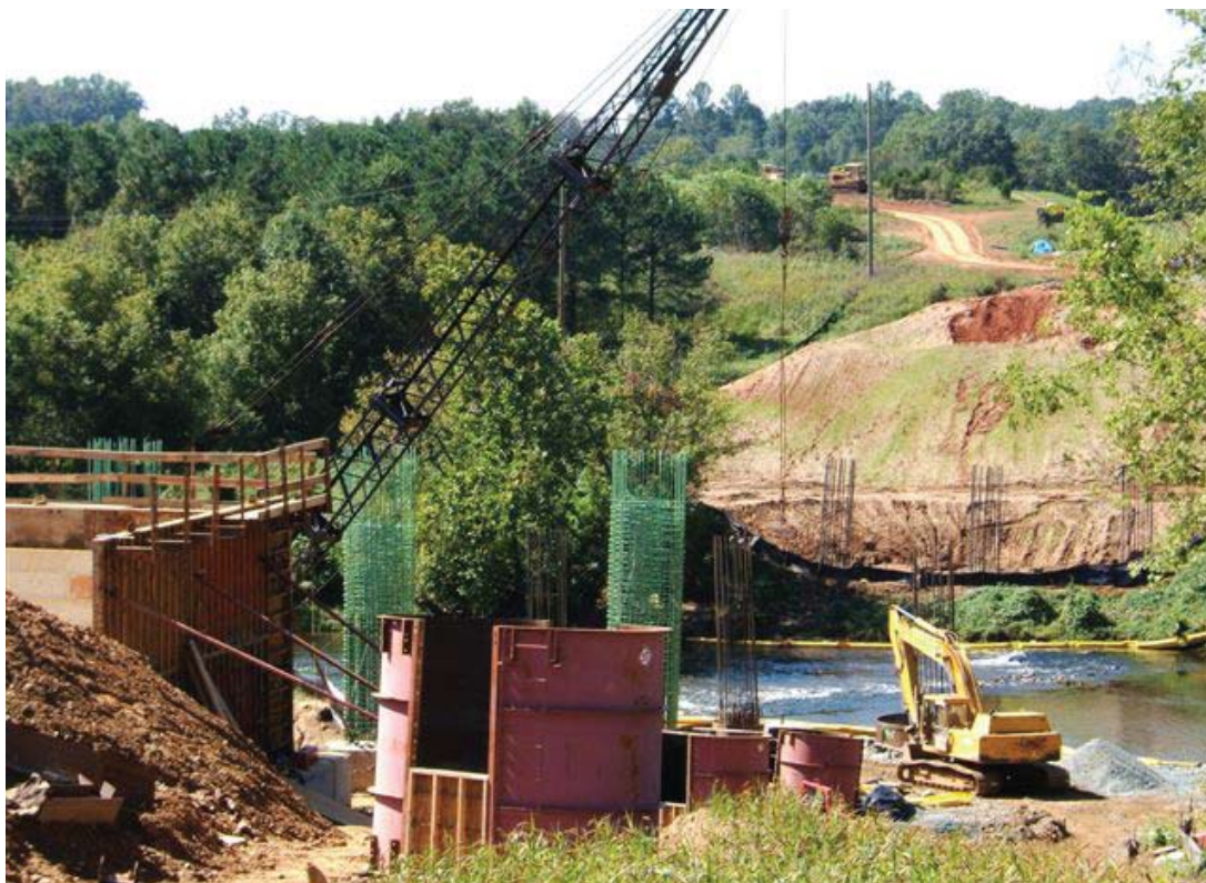
Construction of the new Rivanna Bridge at Palmyra 2006.
