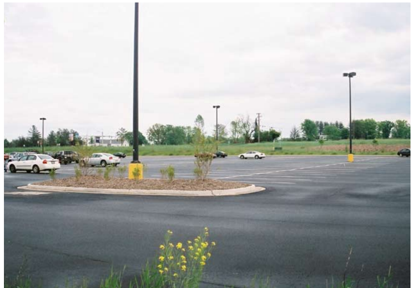
Parking lots are one of the most significant sources of concentrated stormwater runoff.
