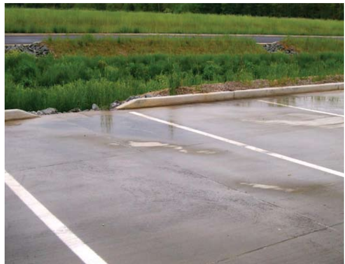
Some water draining off of the parking lot at the Gateway Development in Ruckersville can flow directly into bioswales that absorb some of the runoff and can help filter pollution.
