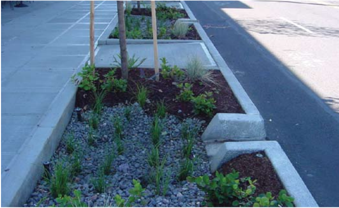
Periodic curb cuts allow some street runoff to drain into planting areas like the ones pictured in the example above. Photo Credit: Lower Columbia River Estuary Partnership.
