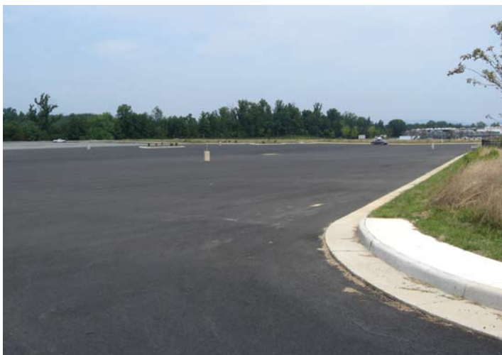
Impervious surfaces from development prevent infiltration of water into the ground and cause stormwater runoff.
