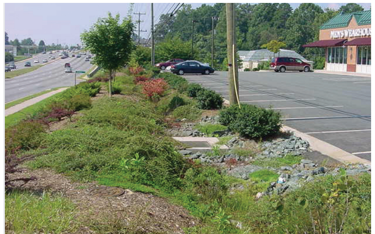
Stormwater that collects on these parking lots at Monticello High School and the Shoppers World Shopping Center flows into vegetated “biofilters” that absorb some of the runoff and help filter out pollutants. During large rainstorms, any excess runoff can spill into overflow drains that usually connect to the storm sewer network.
