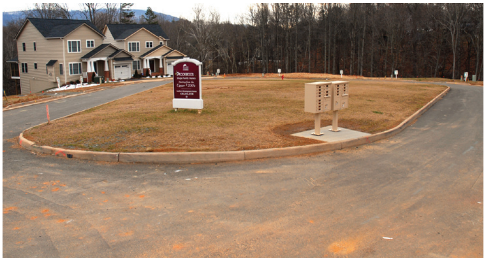
Building landscaped islands in the middle of new cul-de-sacs can help reduce pavement, as seen in this photo of the new Brookwood development currently under construction on Raymond Avenue in Charlottesville. Additional stormwater benefits can be provided if the islands are designed to absorb some runoff from the surrounding street.
