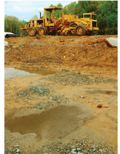
Stormwater runoff can sweep significant amounts of sediment from construction sites into local waterways.
