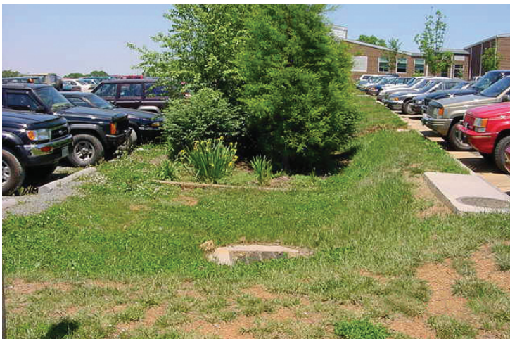
Stormwater that collects on these parking lots at Monticello High School and the Shoppers World Shopping Center flows into vegetated “biofilters” that absorb some of the runoff and help filter out pollutants. During large rainstorms, any excess runoff can spill into overflow drains that usually connect to the storm sewer network.
