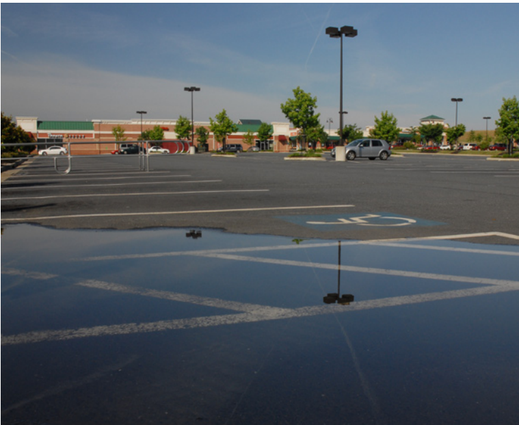
There are still many untapped opportunities for reducing polluted runoff from new parking lots built in the County.
