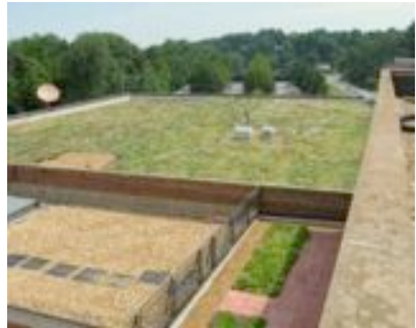
Albemarle County Office Building
