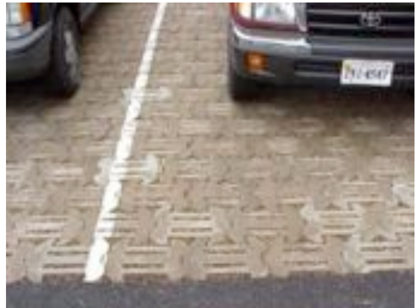
Albemarle County Office Building
