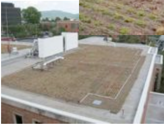
Charlottesville City Hall & Police Building
