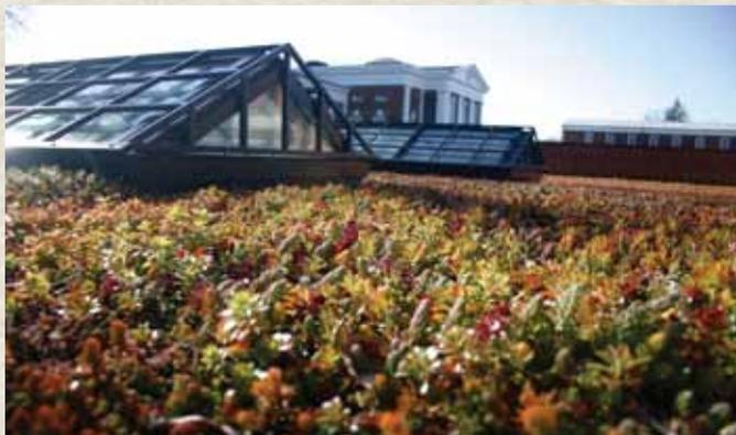
The plants on this green roof at the University of Virginia capture rainfall that would otherwise become stormwater runoff. The green roof also helps reduce heating and cooling needs. Photo/UVa
